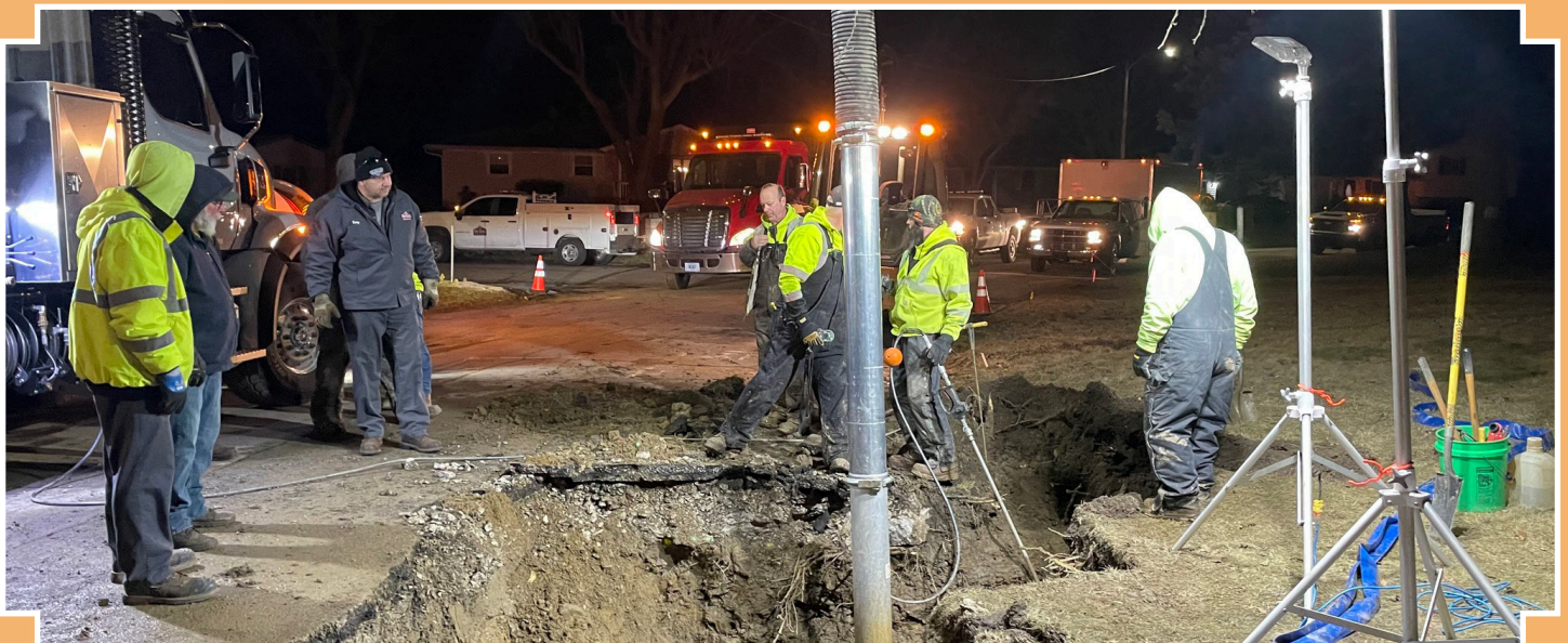
A crew repairs a water main break in Tanglewood
